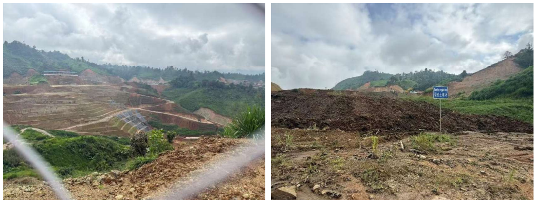
Figure 12.1: Industrial Site Grading
