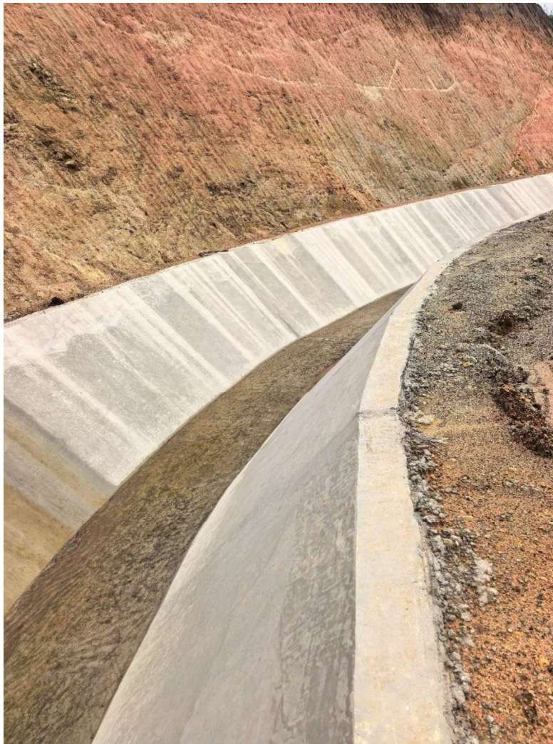
Figure 18.10: As-Built Containment Structures Downstream of the TSF
